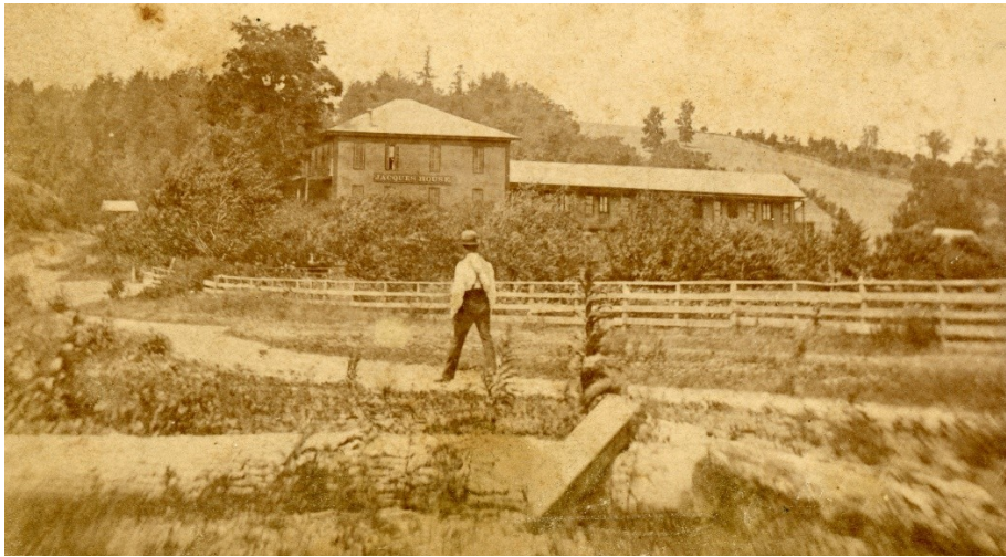
Figure 10 Jacques House looking West
