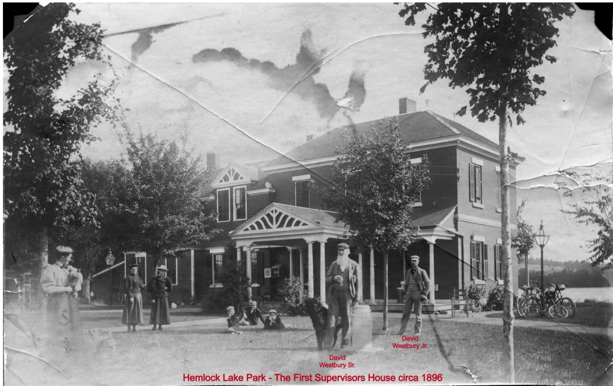
Figure 11 Often incorrectly identified as the "Gate House". It is also called "The Brick"
